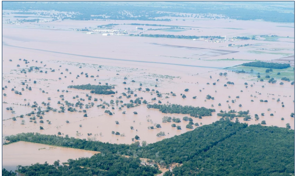
Aerial view of the Ramsey and Terrell units following Hurricane Harvey. (photo courtesy of Brazoria County/Texas DPS)
