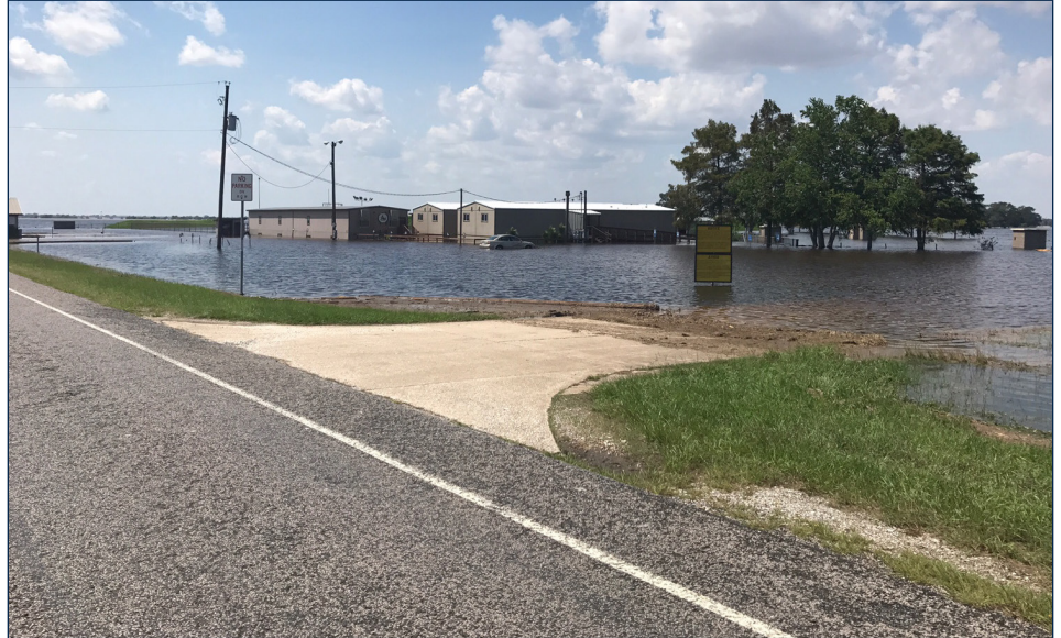
Flooding at the Ramsey Unit.
